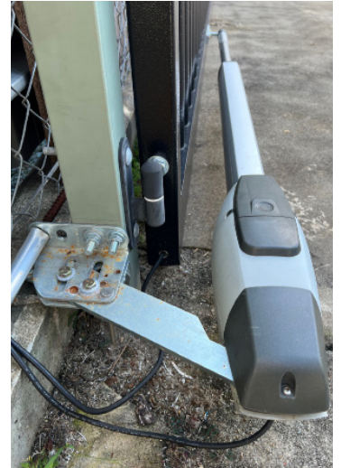
Correct setup showing the arm with an angle to the gate
