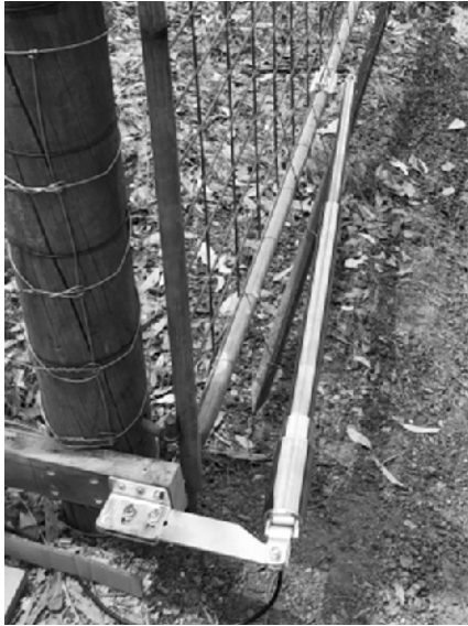
Image above showing rear mounted post bracket with the gate in the open position
