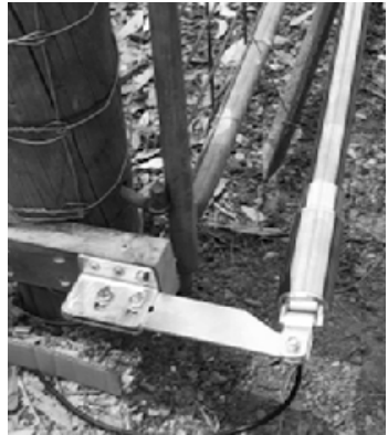
Option A Rear post mounting
