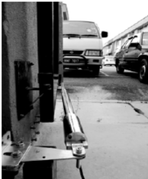
Option B Inside face mounting
