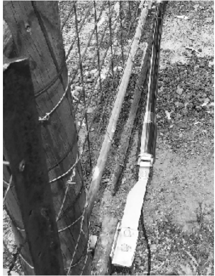
Image above showing rear mounted post bracket with the gate in the closed position
