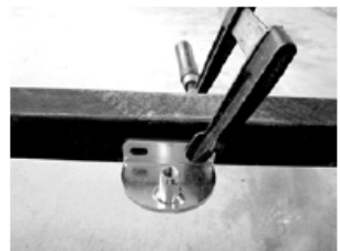
Push-to-Open Gate (Fully Opened) Post bracket mounted on same face as gate hinges
