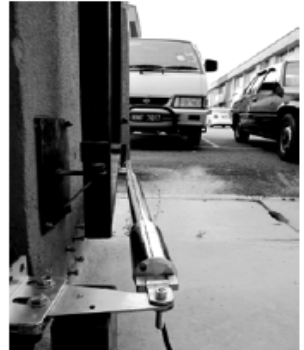
Push-to-Open Gate (Fully Opened) Post bracket mounted on same face as gate hinges
